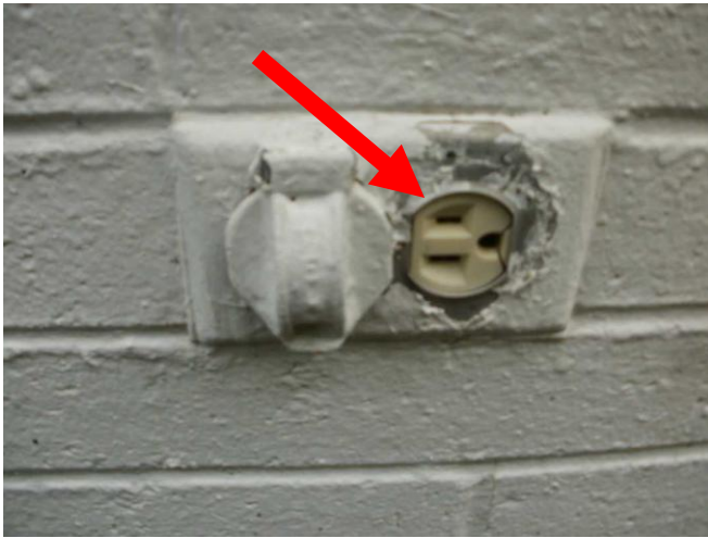
Damaged weather cover.
