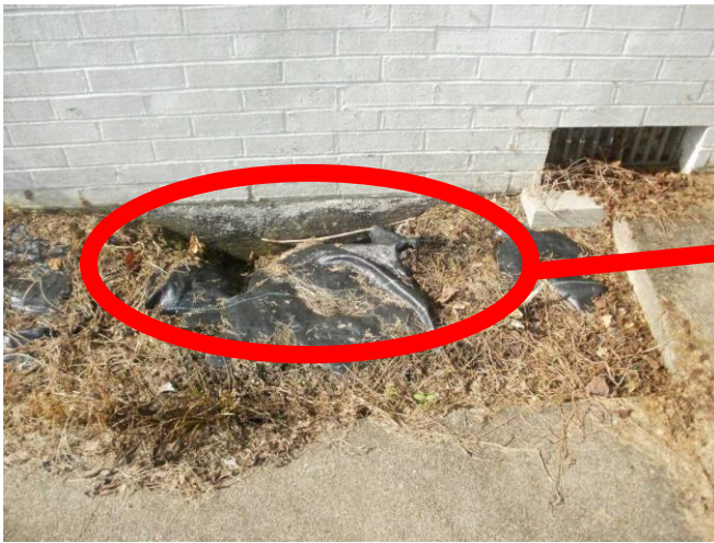
Depression by garage.....Soil erosion at same area of crawlspace. Footer seen.
