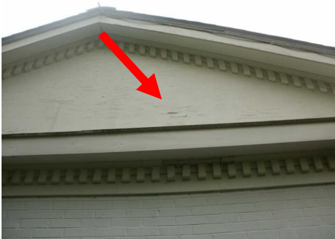
Sample paint peeling at wood areas also.
