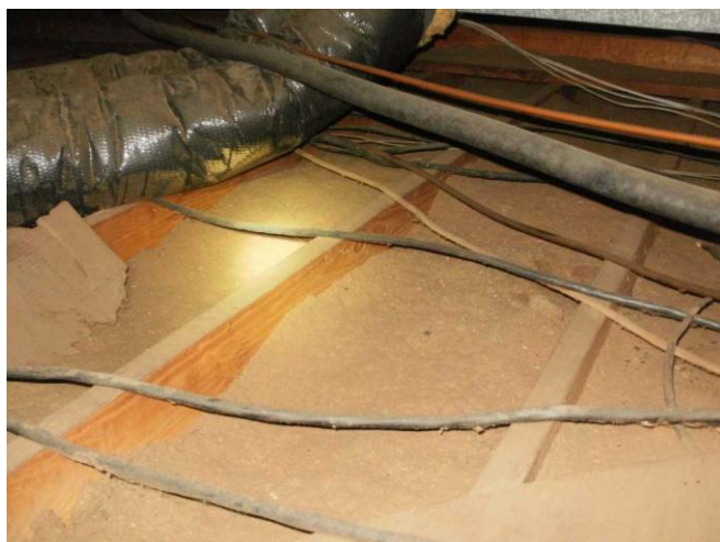
Limited insulation around attic.
