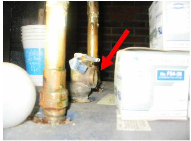
Unit 2 water heater. No t/p drain pipe.
