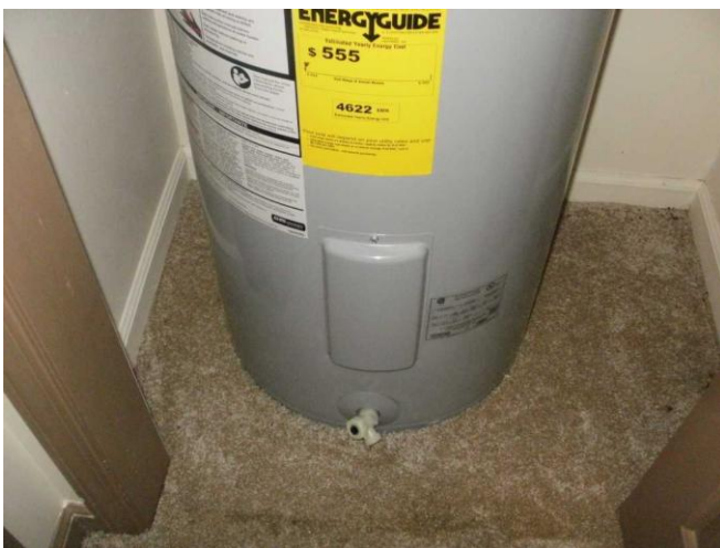
No overflow pan with drain to outside.
