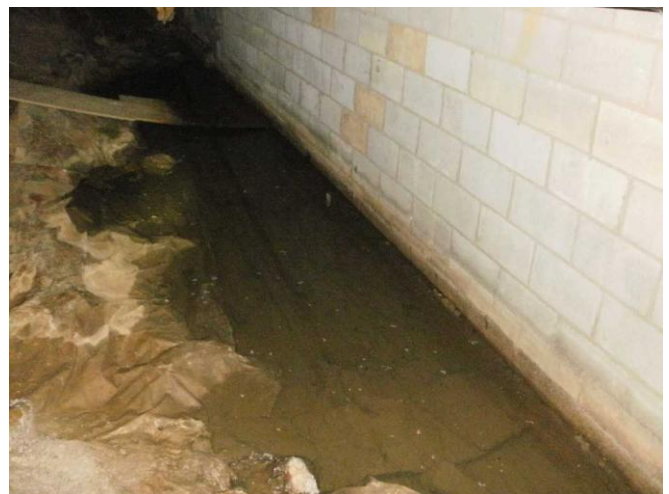
Water standing in left side crawlspace at basement wall... and right side crawl against basement wall.
