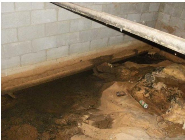
Water standing in left side crawlspace at basement wall... and right side crawl against basement wall.
