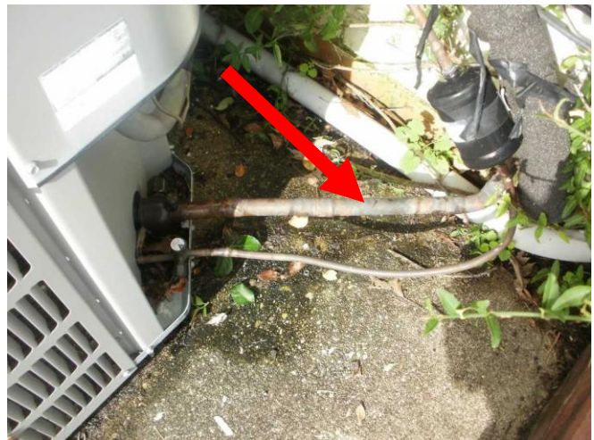
Sample maintain line set insulation both units.....
