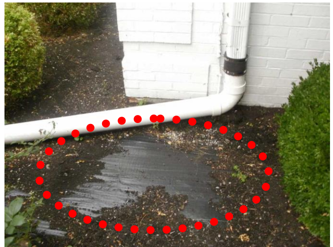
Signs of ponding around house.
