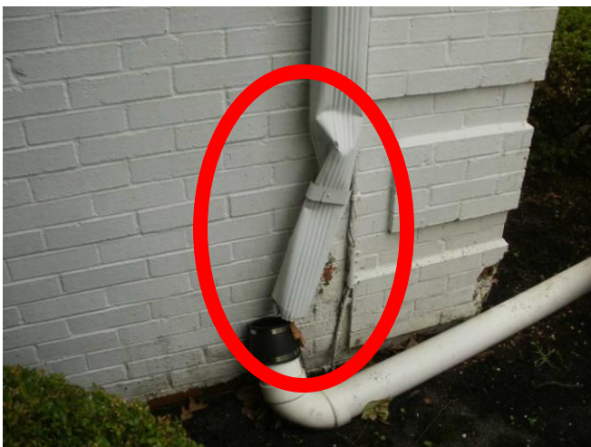
Drain pipe disconnected.
