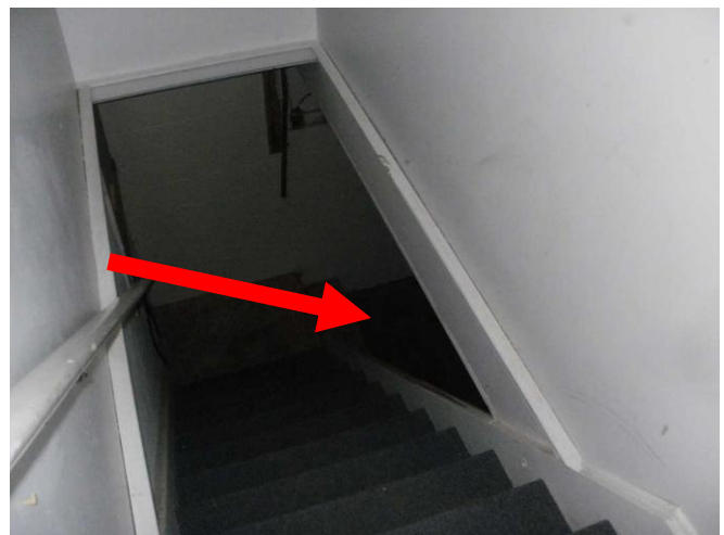
Open railing to basement.
