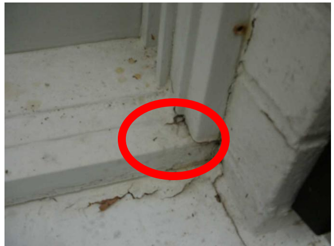
Sample window sill and trim damages.
