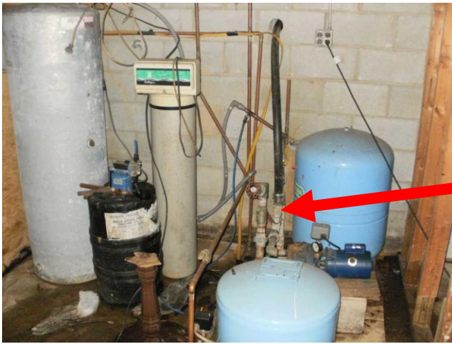
Pressure tank, pump and softener.
