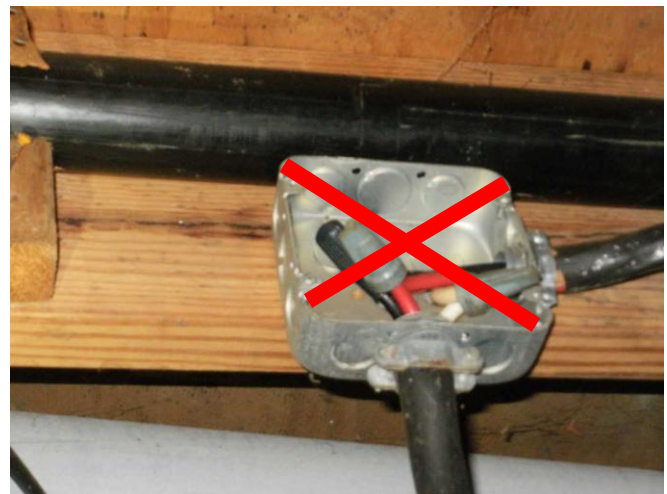
Missing cover plate in basement.
