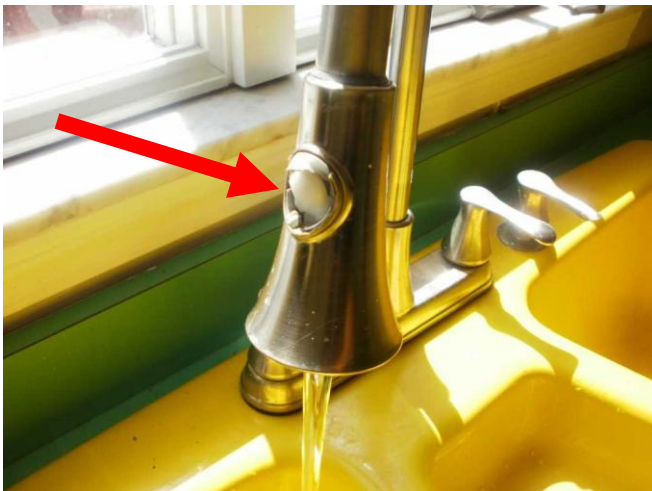
Sink sprayer button damaged.
