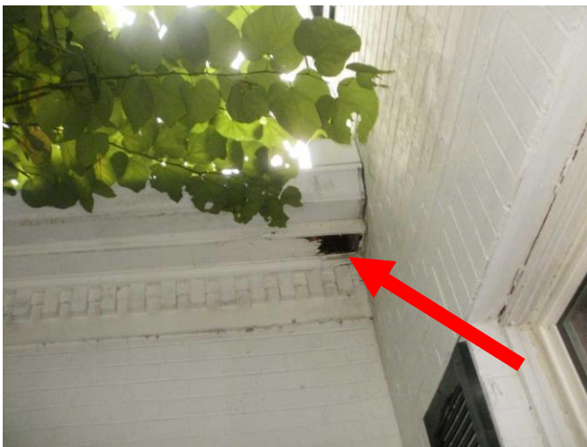
Sample damaged soffit by garage.....and at rear.
