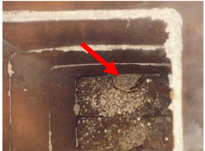
Sample visible nesting in chimney.
