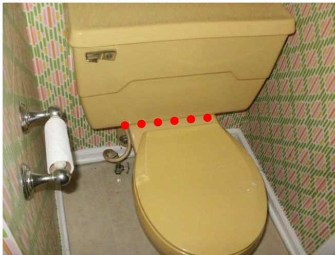
Toilet tank to bowl leaking.
