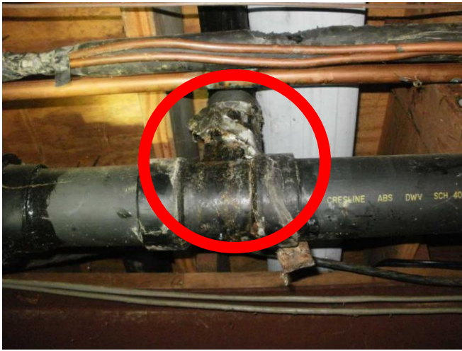
Duct tape repairs on drain line.
