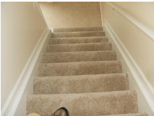
Steep steps at rear hall and shallow treads.
