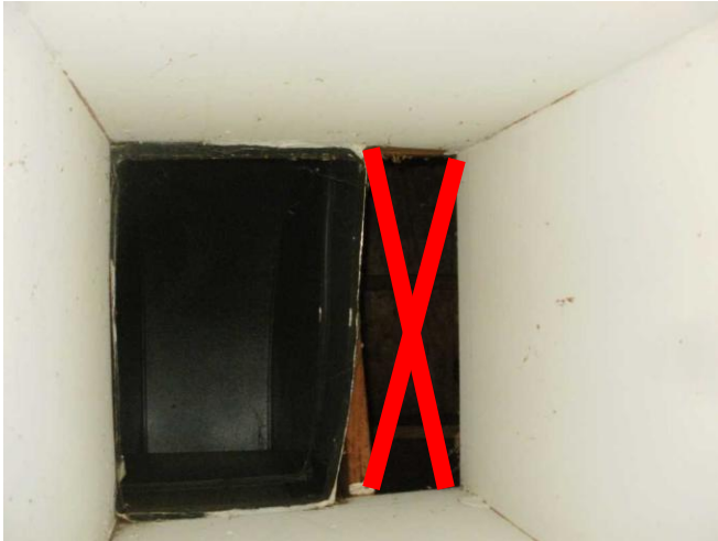
Laundry chute closet missing ceiling areas.
