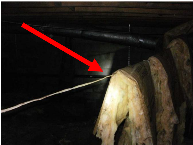
Some wires are not secured and are holding insulation.
