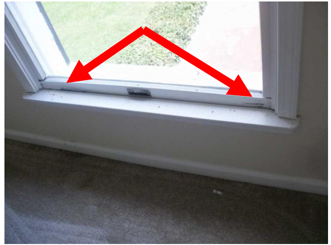
Sample sash damage at old wood windows.....Areas visible inside.
