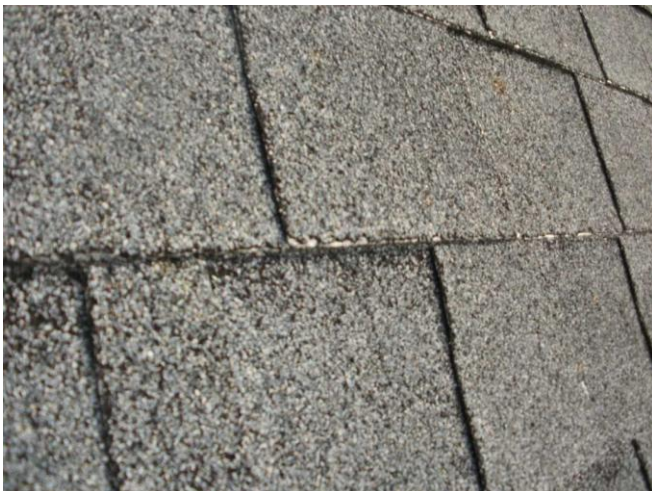
Up close of shingle wear.....Sample larger area above master bedroom.
