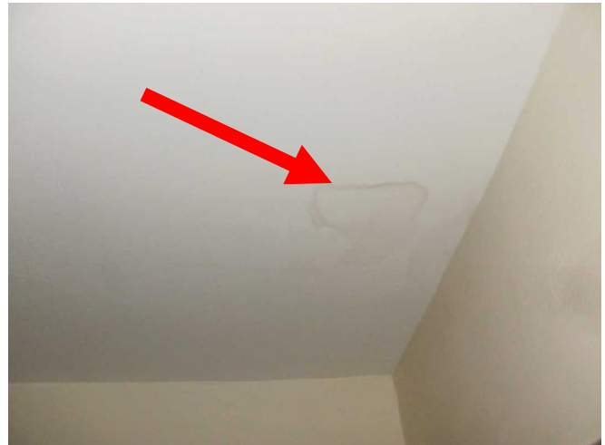
Damp staining on ceiling by water heater closet.
