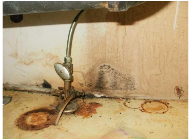
Sample bio growth under sink.
