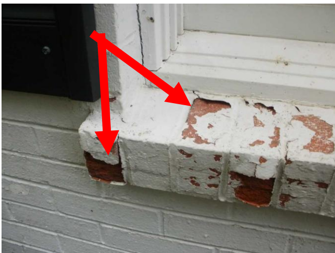
Sample paint issues and brick damage.....various areas.
