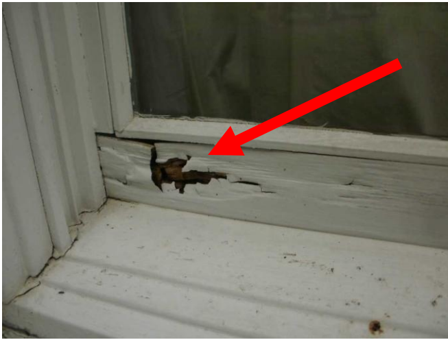
Sample sash damage at old wood windows.....Areas visible inside.
