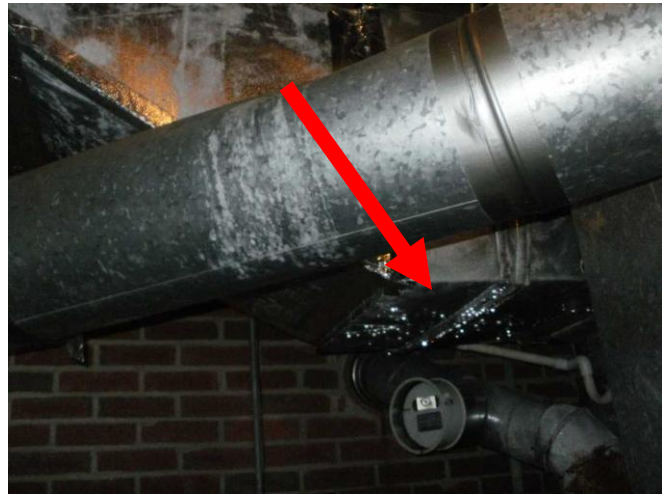
Water coming from evap coil area of unit 1.
