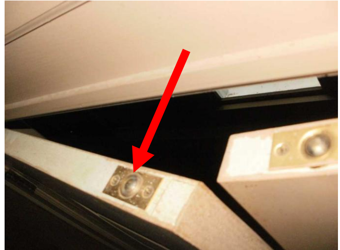
Door ball assembly damaged. (replaceable part)
