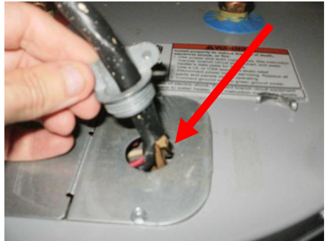
Unit 1 water heater romex concern.
