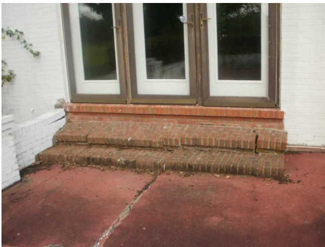
More step height issues, settlement and damage.....
