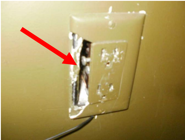
Damaged cover plate in office.
