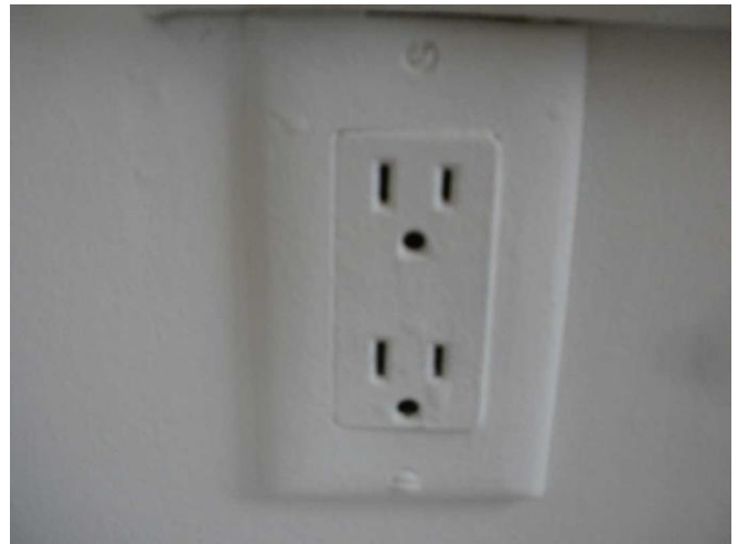
Sample outlets painted over or not tested. (Tight fitting)
