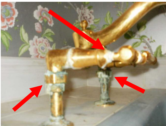
Leaking concerns at bath 1 tub controls.
