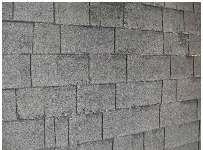
Up close of shingle wear.....Sample larger area above master bedroom.
