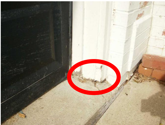
Door frame damaged wood.
