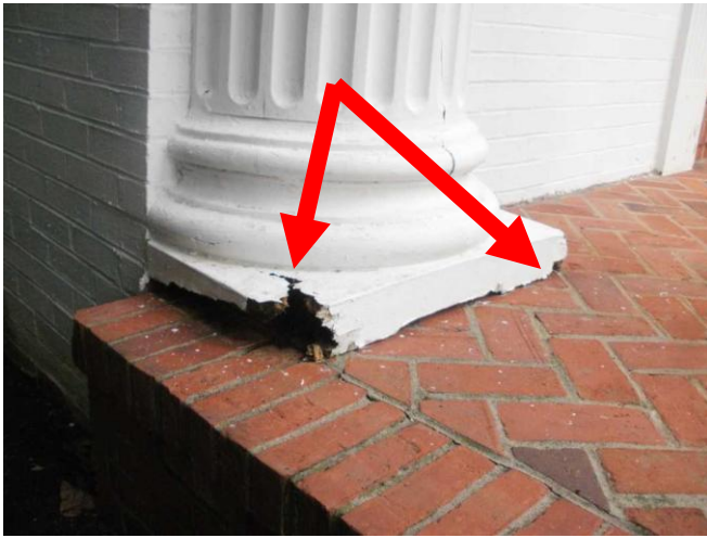
Damaged wood at pillars and trim against house.....Samples.
