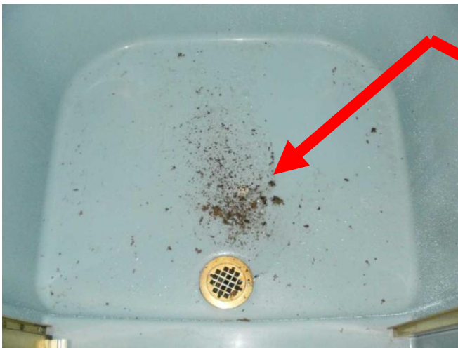
Stuff in bath 1 shower and tub from recessed lights.....No trim kits.
