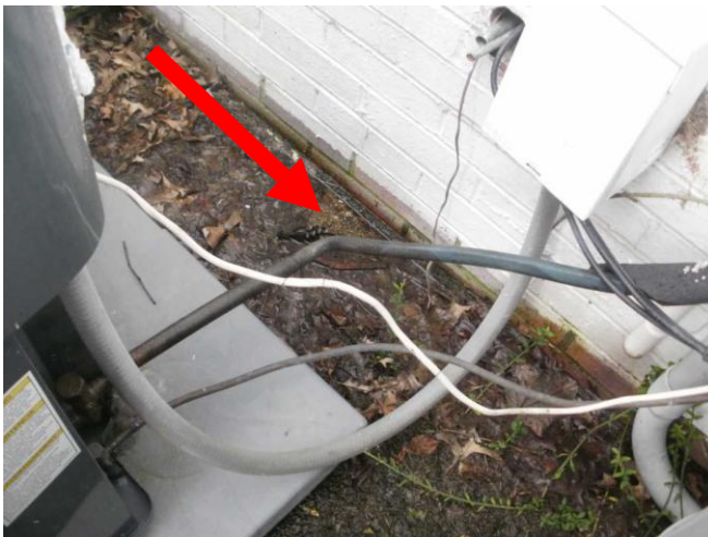
Sample maintain line set insulation both units.....
