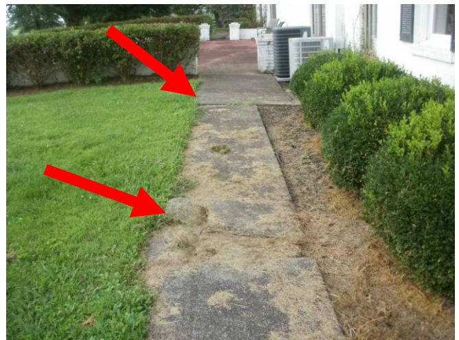
Sample cracked sidewalks and more sloping.
