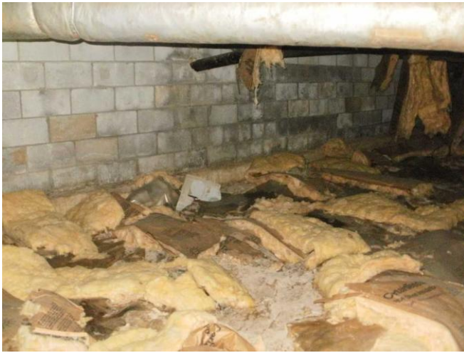
Sample insulation has fallen down. Signs of damp walls.
