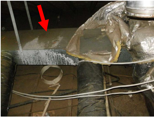
Trunk in attic not insulated and sweating. Sample.
