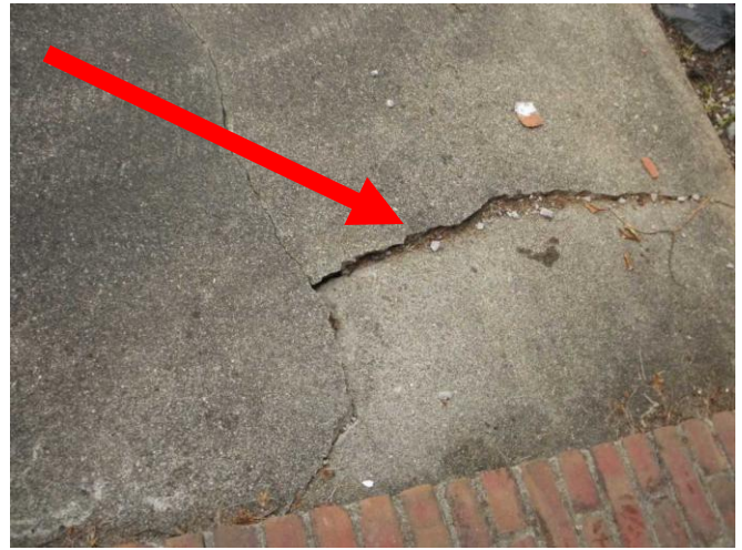
Outside patio at office settled and cracked.
