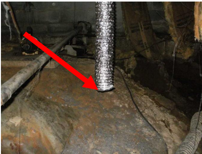
Dry vents to crawlspace.
