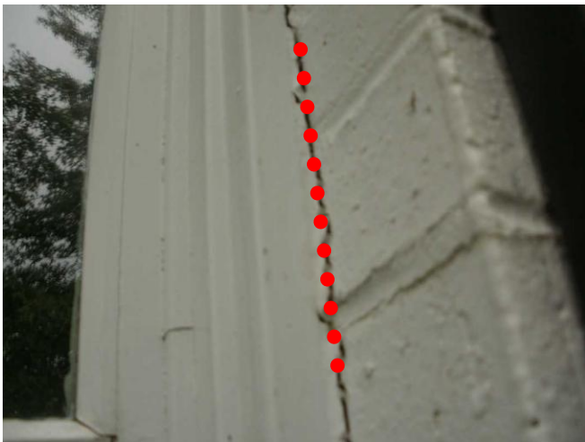
Sample sealant around windows to brick.
